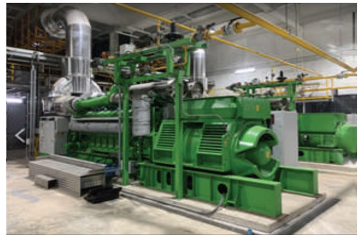
Exhibit 7: Gas engine and generator
