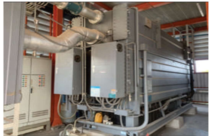
Exhibit 8: Absorption chiller
