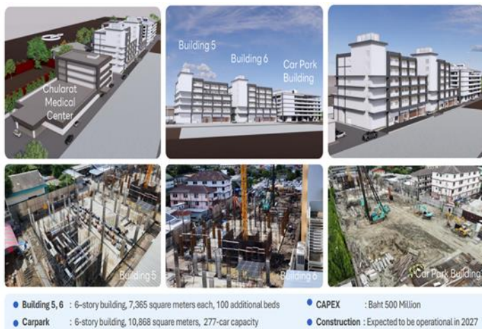
Exhibit 79: Chularat 3 Hospital's facility extension
