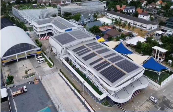
Exhibit 5: The 2.04 MW rooftop solar energy system
