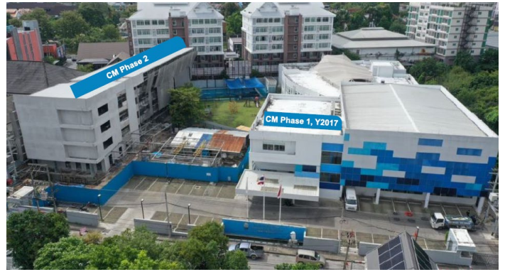
Exhibit 2: CM phase 2 construction update (+300 seats)
