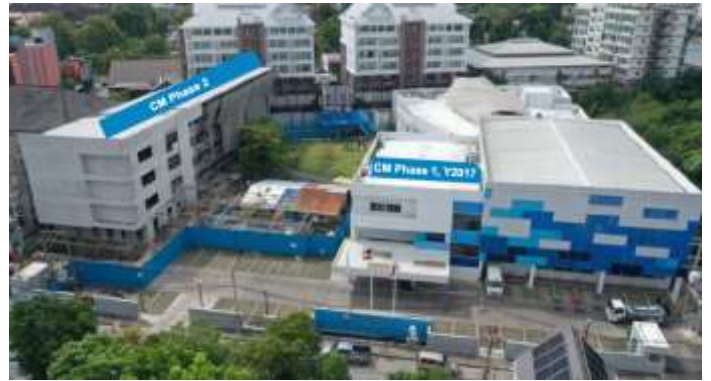
Exhibit 2: CM phase 2 construction update (+300 seats)
