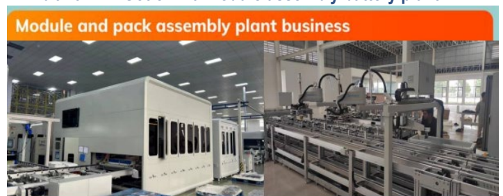
Exhibit 16: NV Gotion – a module assembly battery plant
