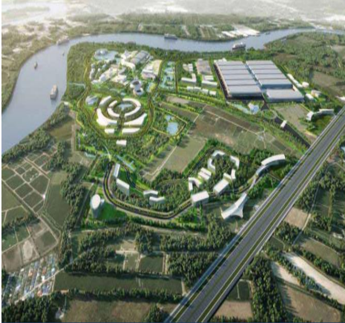
Exhibit 9: Blue Tech City Industrial Estate aerial view
