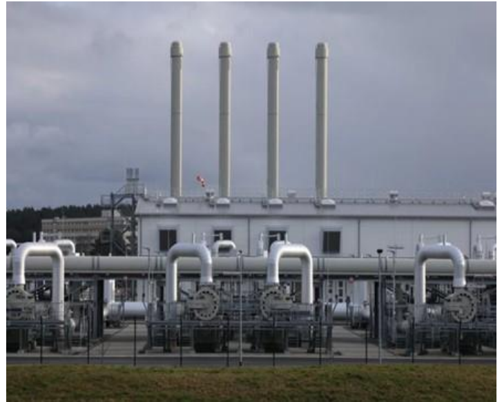
Exhibit 36: The receiving station of the Nord Stream 2 gas pipeline stands near Lubmin, Germany
