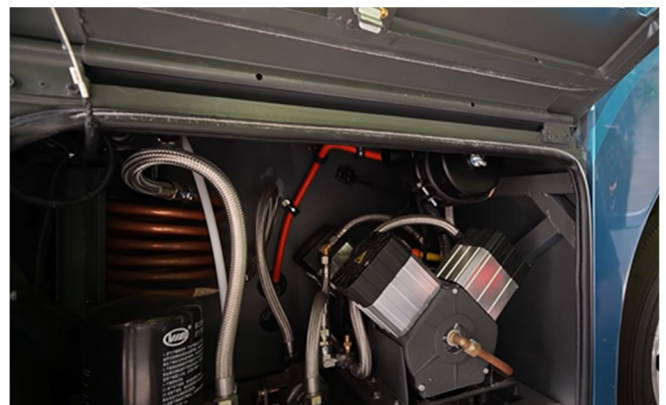
Exhibit 4: Battery-installed in e-bus (350kWh)
