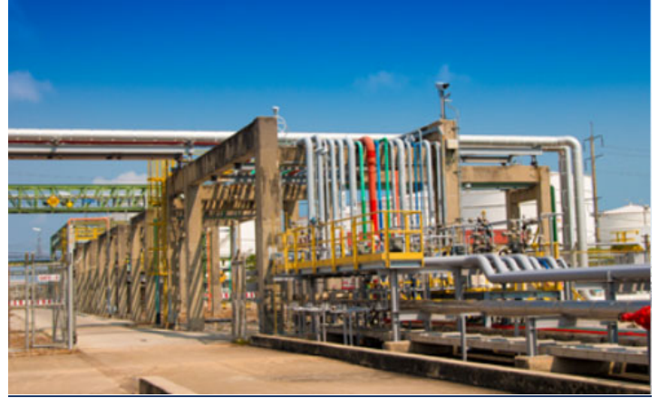
Exhibit 2: Oil pipeline at the refinery
