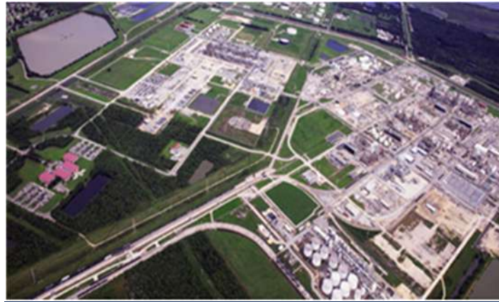
Exhibit 7: IOD site aerial view
