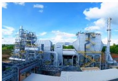
Exhibit 7: Flue gas cleaning at CV
