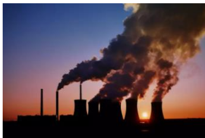
Exhibit 58: Japan's JERA coal-fired power plant
