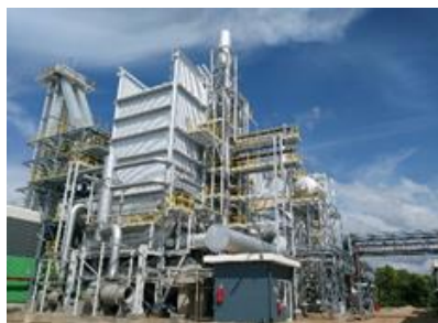
Exhibit 7: Flue gas cleaning at CV
