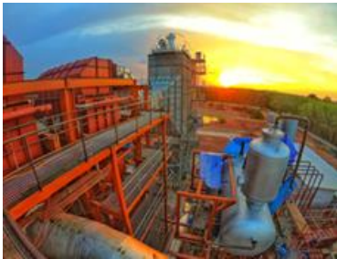
Exhibit 16: Boiler at RTB
