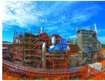
Exhibit 17: Flue gas cleaning at RTB
