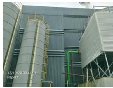
Exhibit 20: Water treatment & cooling tower at CPX
