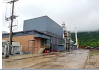
Exhibit 11: Control room & turbine hall at CPL
