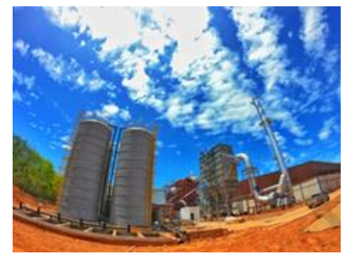
Exhibit 18: Water treatment at RTB
