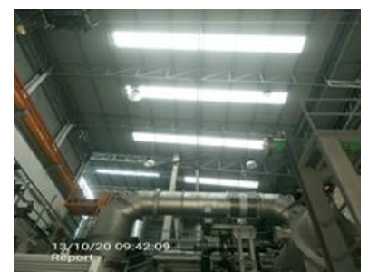
Exhibit 21: Turbine & generator at CPX
