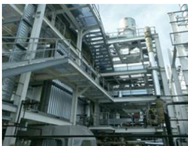
Exhibit 19: Boiler at CPX
