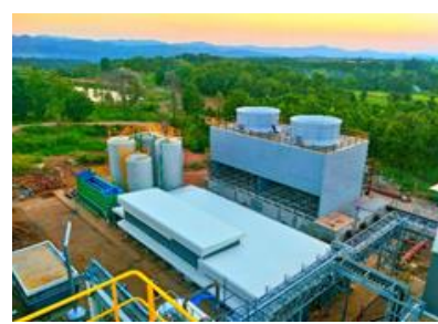
Exhibit 6: Water treatment & cooling tower at CV
