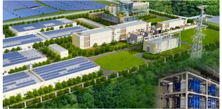
Exhibit 4: Microgrid energy storage system
