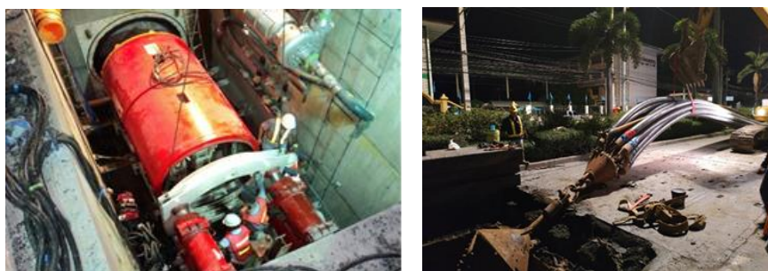
Figure 8: Pipe Jacking & Horizontal Directional Drilling
