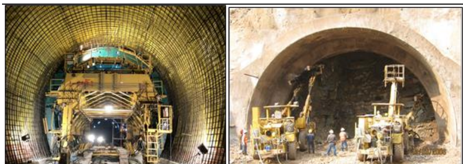
Figure 2: Tunnel & Shaft works
