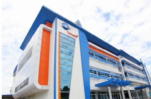
Figure 5: Interlink Data Center
